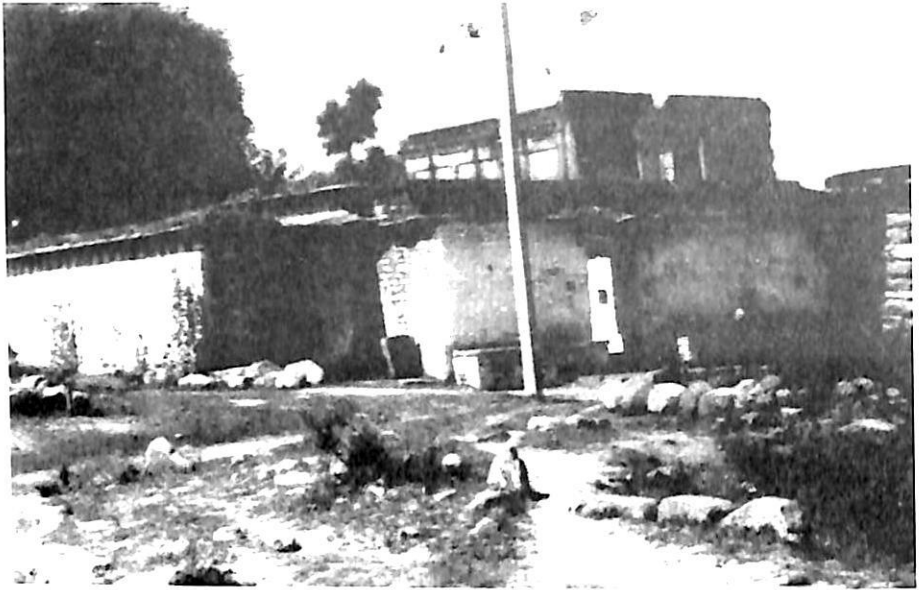
The dilapidated house at Surabhi built in 1886-87
